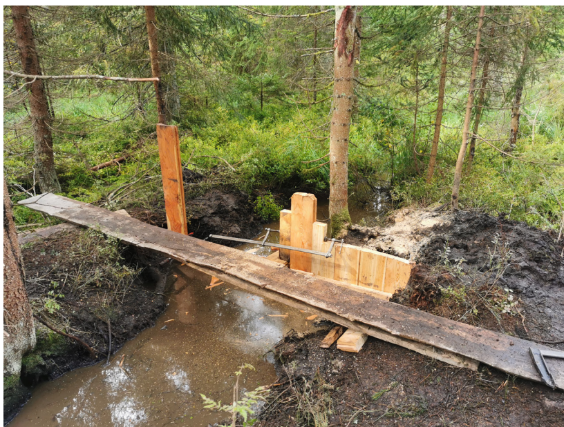
Figure 3 Construction of a sheet pile wall in a peatland in the German Erzgebirge (Photo: L Wagner)
